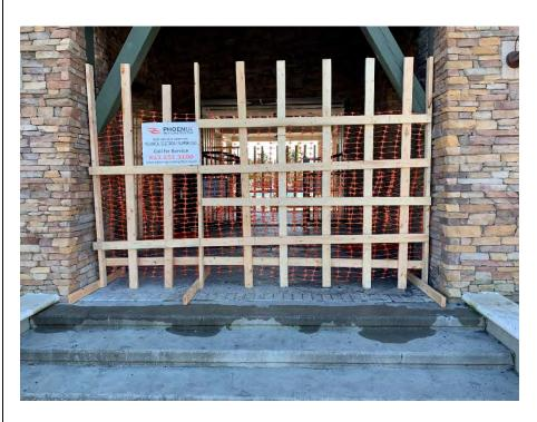
There was a fire at the entrance of the amenity center. It will remain blocked off until repairs are complete. There was damage to the ceiling, stone, light fixtures, electrical wiring, and tile.
